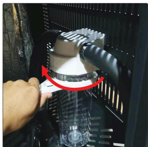
Remove the filter using a special wrench
